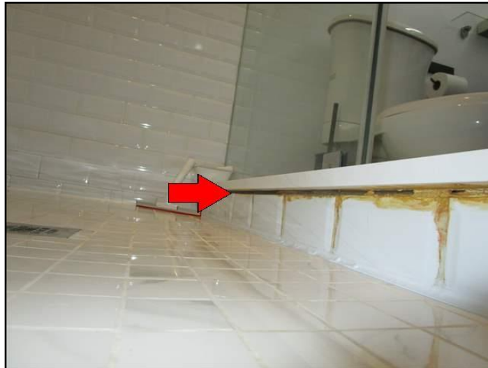
Grout loose, missing or deteriorated
