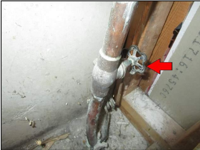
Main water shut-off valve
