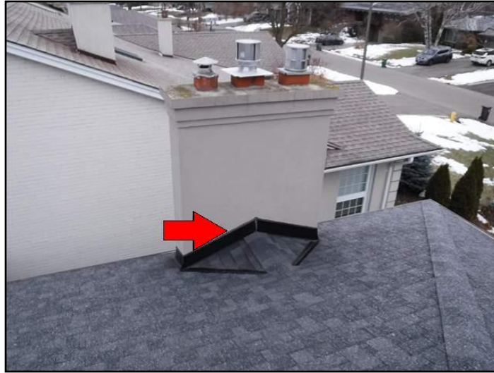
Caulking deteriorated/ineffective
