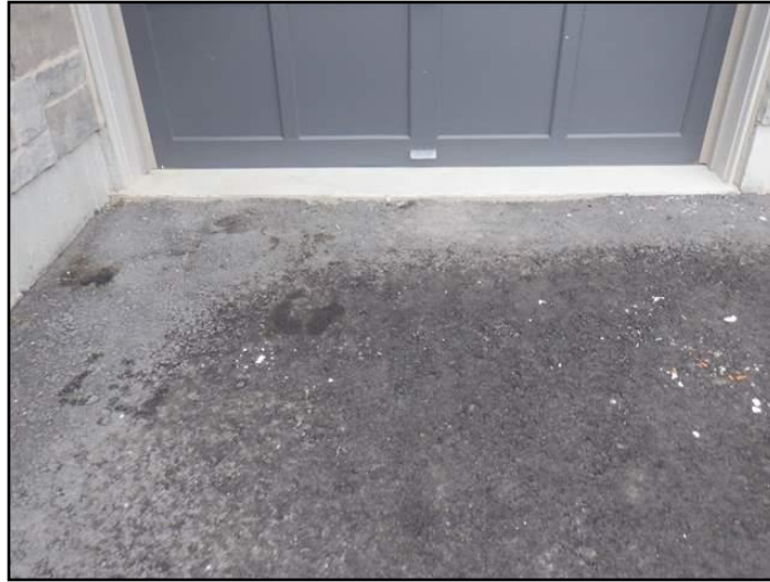
Top asphalt layer not yet applied
