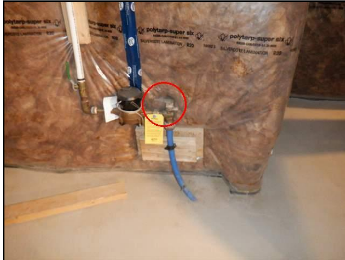
Main water shut-off valve
