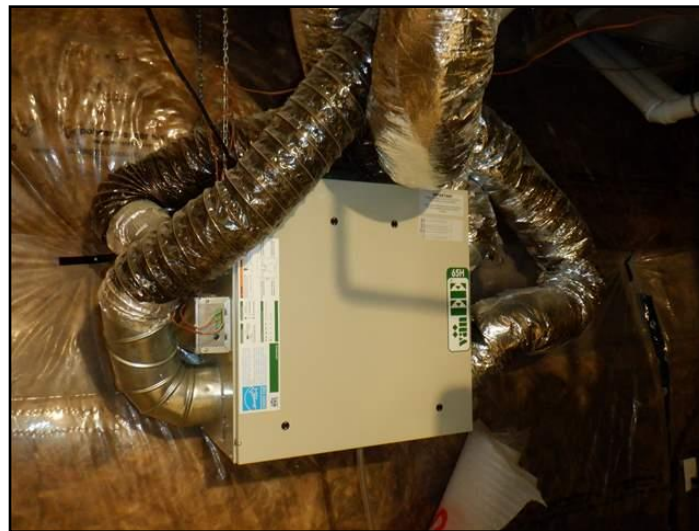
Heat recovery ventilator (HRV)
