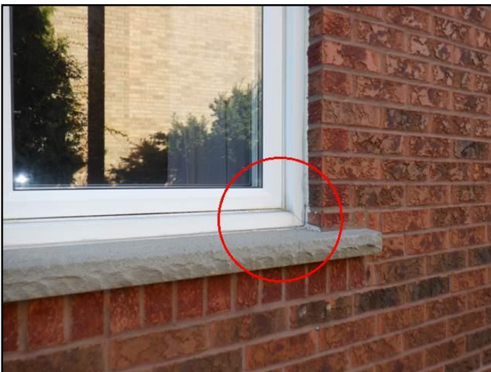
Example: Caulking deteriorated. Sill cracked
