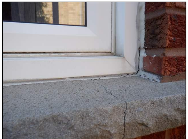
Example: Caulking deteriorated. Sill cracked
