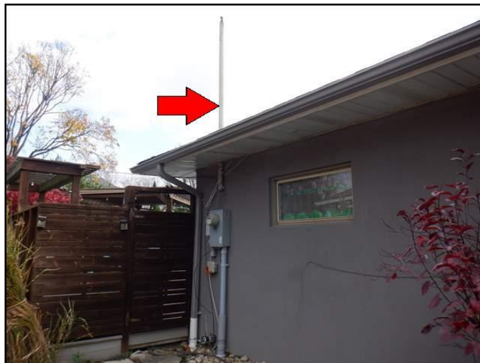
Abandoned mast should be removed
