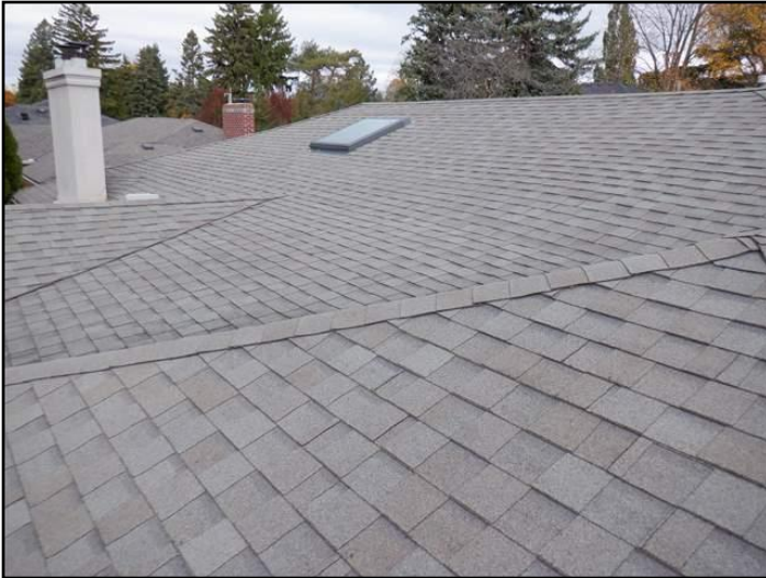
Asphalt shingles
