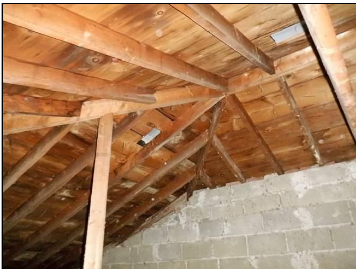
Rafters/roof joists
