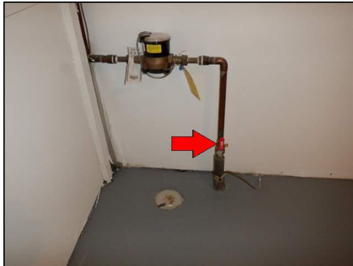
Front of the basement
