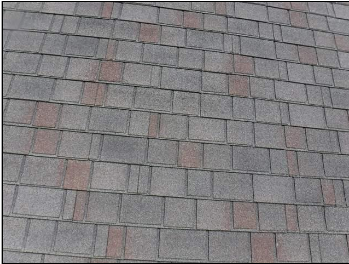
Asphalt shingles
