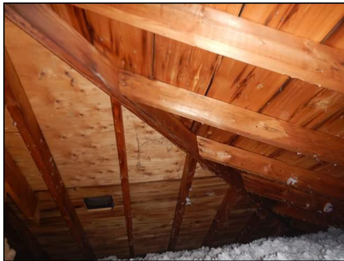
Rafters/ceiling joists
