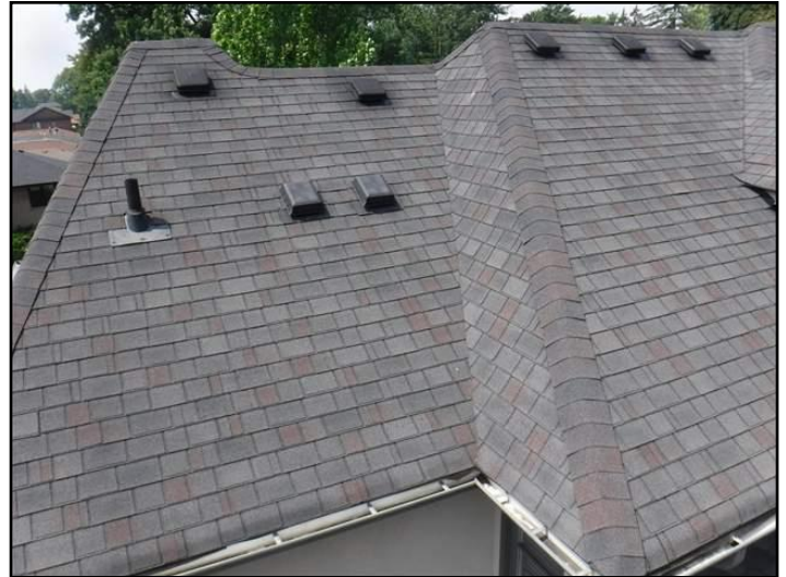
Asphalt shingles
