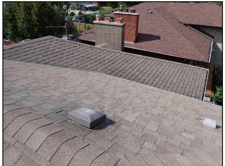
Shingles are in good/aging condition
