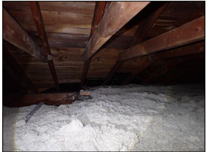
Insulation is evenly distributed
