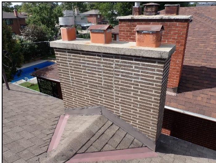
Chimney is in good condition
