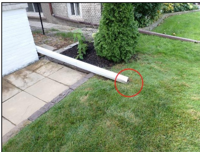
Maintain discharge well away from foundation
