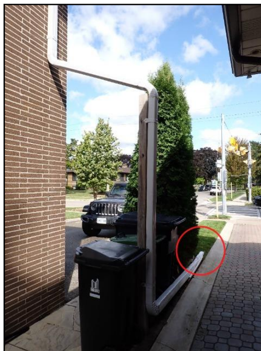
Maintain discharge well away from foundation
