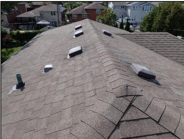
Shingles are in good/aging condition
