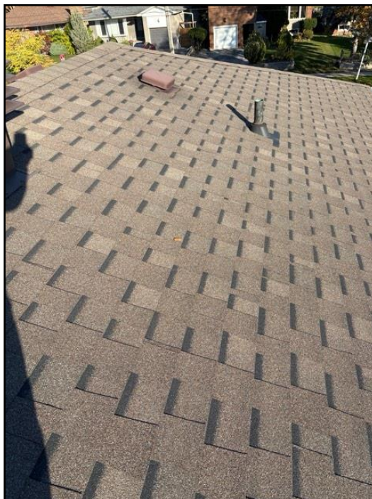
Asphalt shingles
