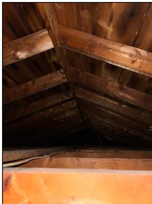
Rafters/roof joists
