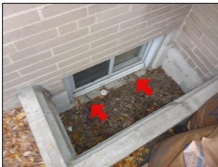
Window close to grade in well
