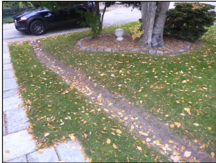
Gully at front to control drainage
