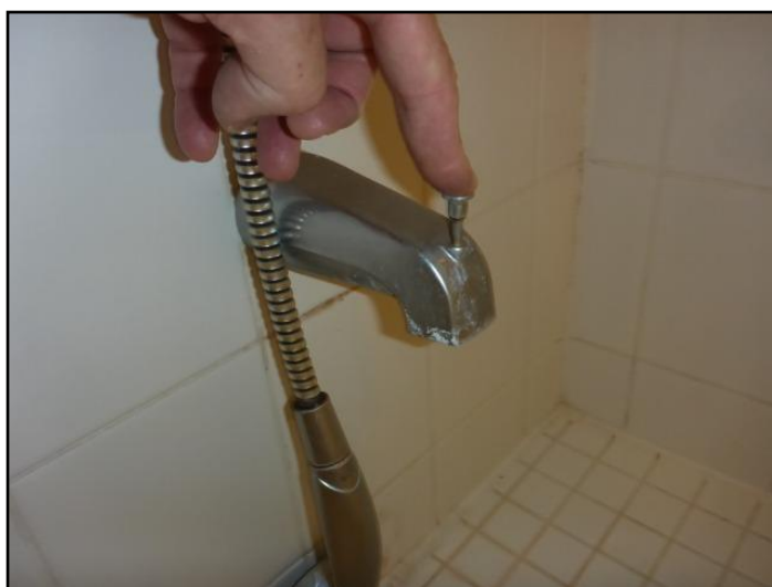
Shower diverter stuck in "up" position
