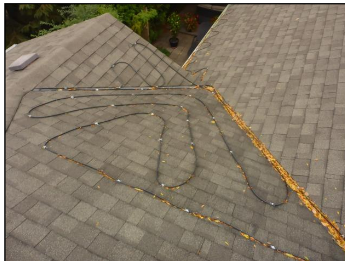
Ice melt cables noted at rear roof
