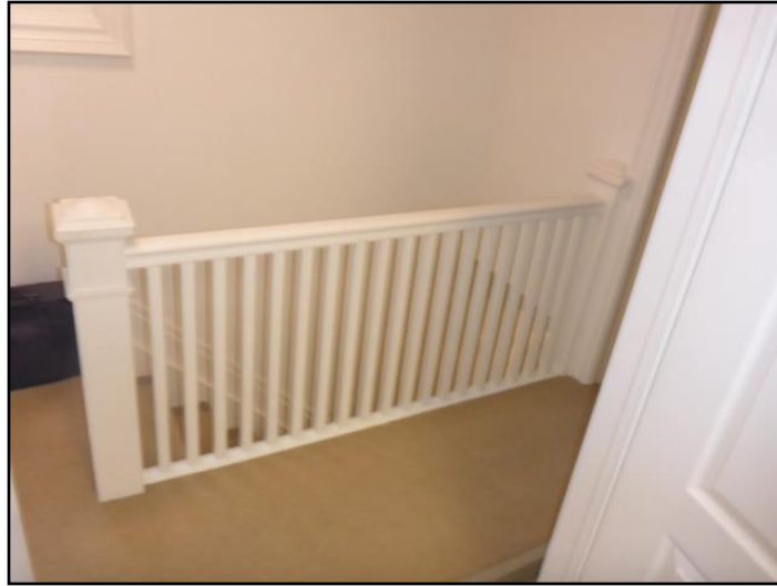
Low railing at hallway
