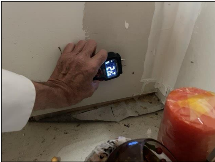
Right Side under Stairs
