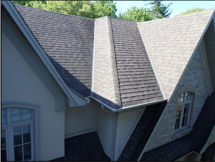
Asphalt shingles
