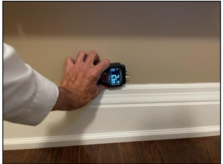
Left side Electrical room
