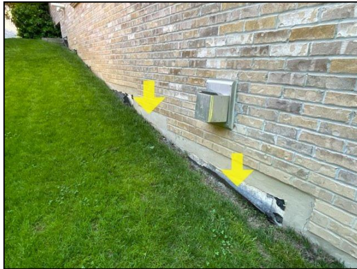
Evidence of water proofing
