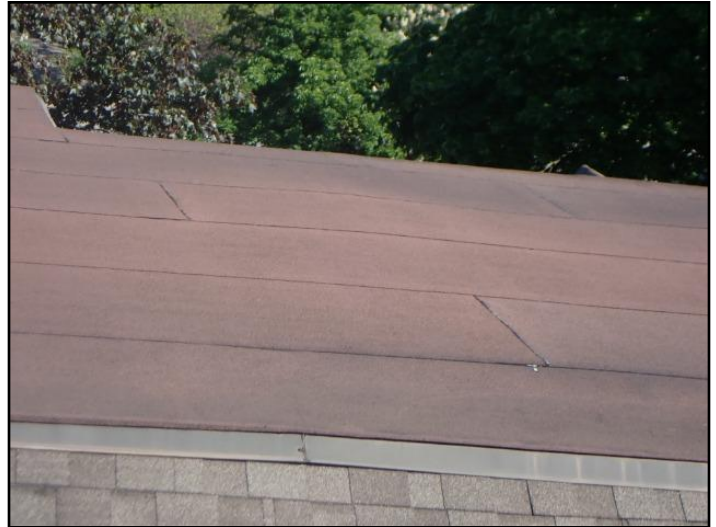
Modified bitumen membrane
