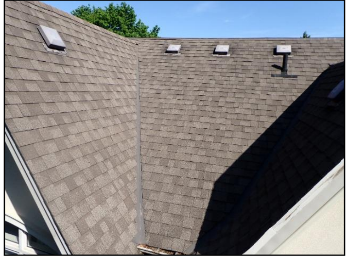
Asphalt shingles
